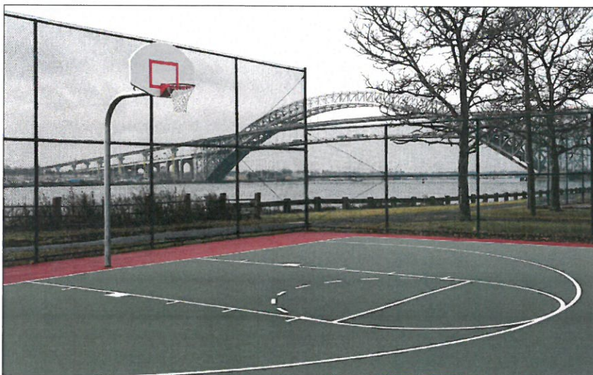
In the shadow of the Bayonne Bridge, PPG excavated 7,300 tons of soil and debris at Dennis Collins Park and replaced one basketball court.
